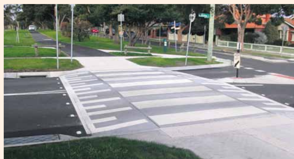
A new zebra crossing has been constructed in Narrawong Road, Caulfield South. Photo: Glen Eira City Council's Transport Planning Department.
