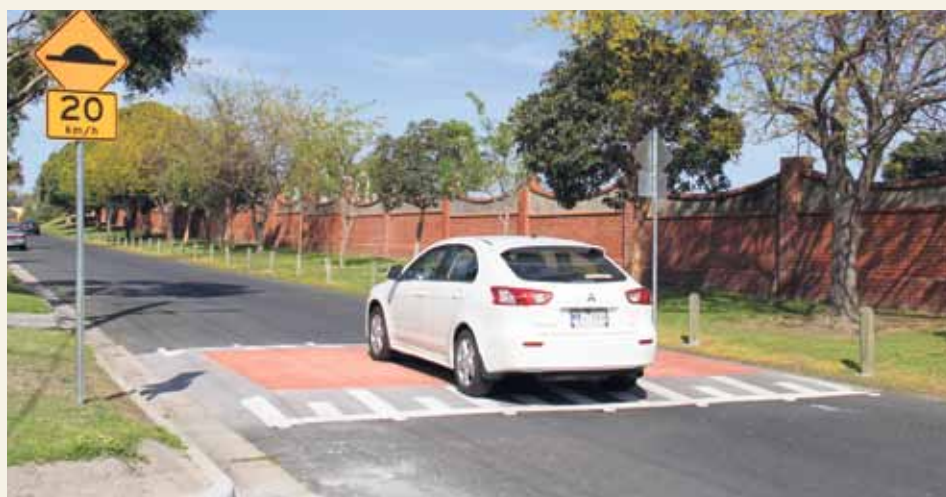
Council has constructed two road humps in Sheffield Street, Caulfield South to reduce vehicle speeds. Photo: Belinda Foley.
