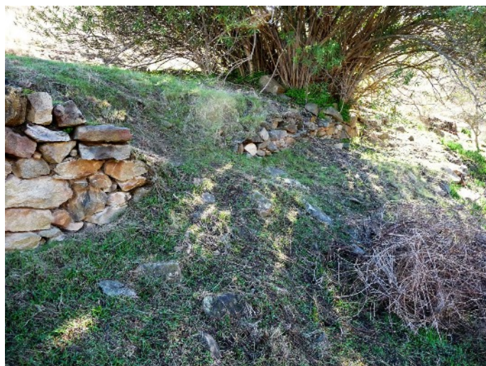
This wall was undermined by rabbits and overwhelmed by cattle. There was enough of the old wall remaining to establish the style and dimensions.
