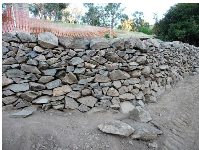
Much of the original large filler stone was used to complete the face of the wall
