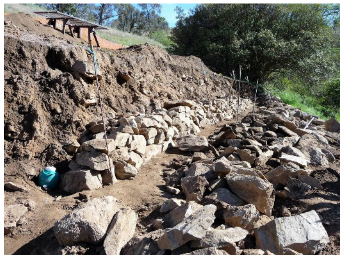
The wall (previous page) was stripped out and rebuilt with the original stone
