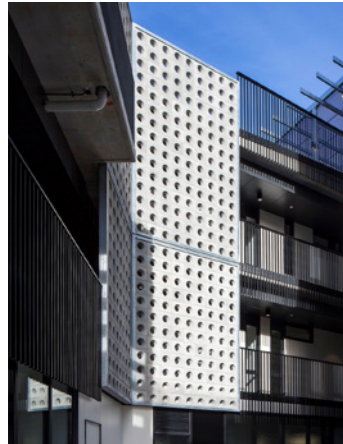
Breezeblock for open-air ventilation in car park.
