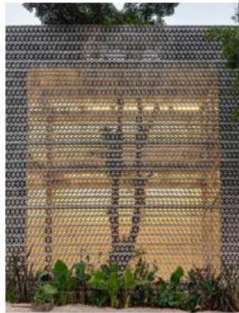
Breezeblock for open-air ventilation in car park.
