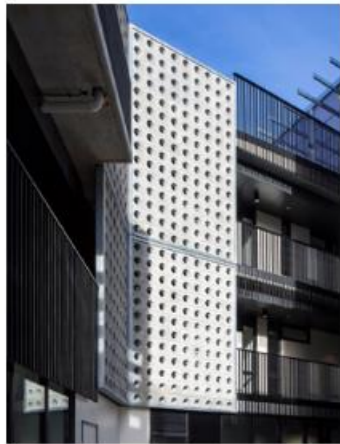
Breezeblock for open-air ventilation in car park.
