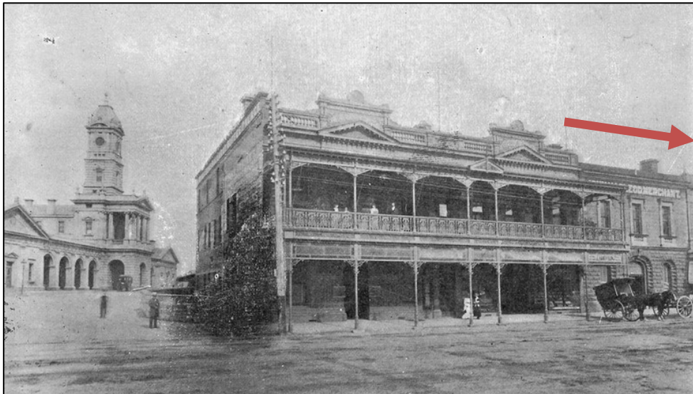
Figure 24 Undated image of Reid's Coffee Palace, with the railway complex to the left and the subject buildings to the right indicated by the red arrow. This key historic view of the Ballarat Railway Station from Lydiard Street will be unchanged by the proposal. Source: Victorian Collections
