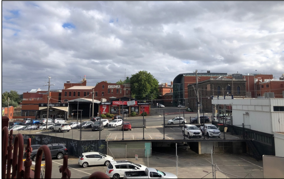
Figure 19 View south towards Mair Street from the top of the railway embankment.
