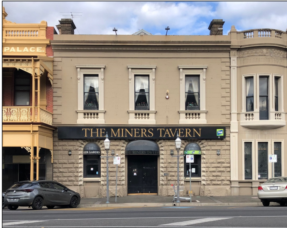
Figure 9 The Lydiard Street frontage of the former warehouse at 122 Lydiard Street.
