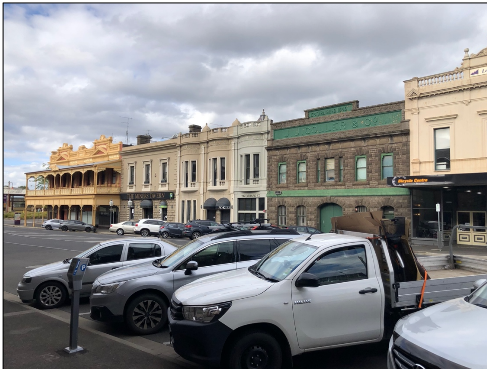
Figure 14 View of the east side of Lydiard Street from the south-west.
