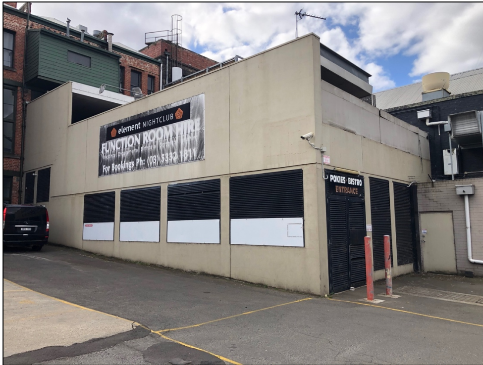
Figure 12 Modern addition at the rear of the shops at 116-118 Lydiard Street.
