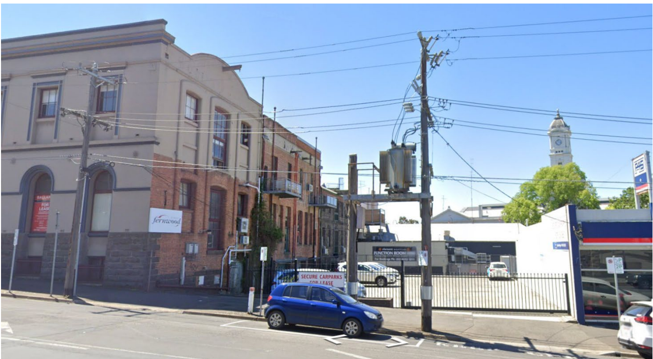
Figure 11. No. 104-110 Lydiard Street South, and No. 114 -116 Lydiard Street North (rear from Mair Street)
