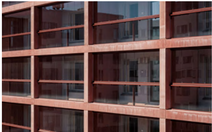
Expressed concrete grid with recessed glazing.
