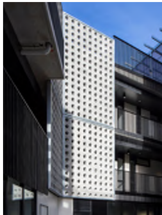
Breezeblock for open-air ventilation in car park.
