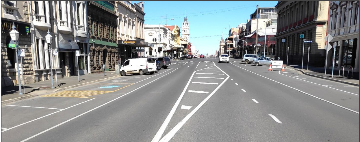
Figure 2.3 Lydiard Street (facing south to Mair Street intersection)
