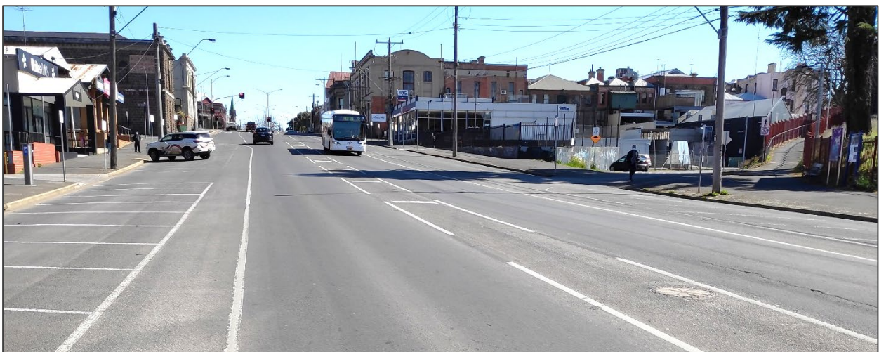
Figure 2.4 Mair Street (facing west towards site)
