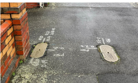
Figure 8 Existing communications infrastructure in Humffray St footpath
