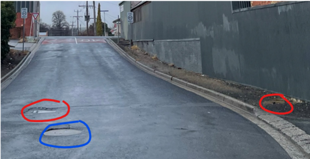
Figure 12 Existing water authority assets in Porter Street
