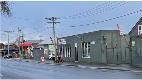
Figure 6 Existing overhead services connections on Humffray Street
