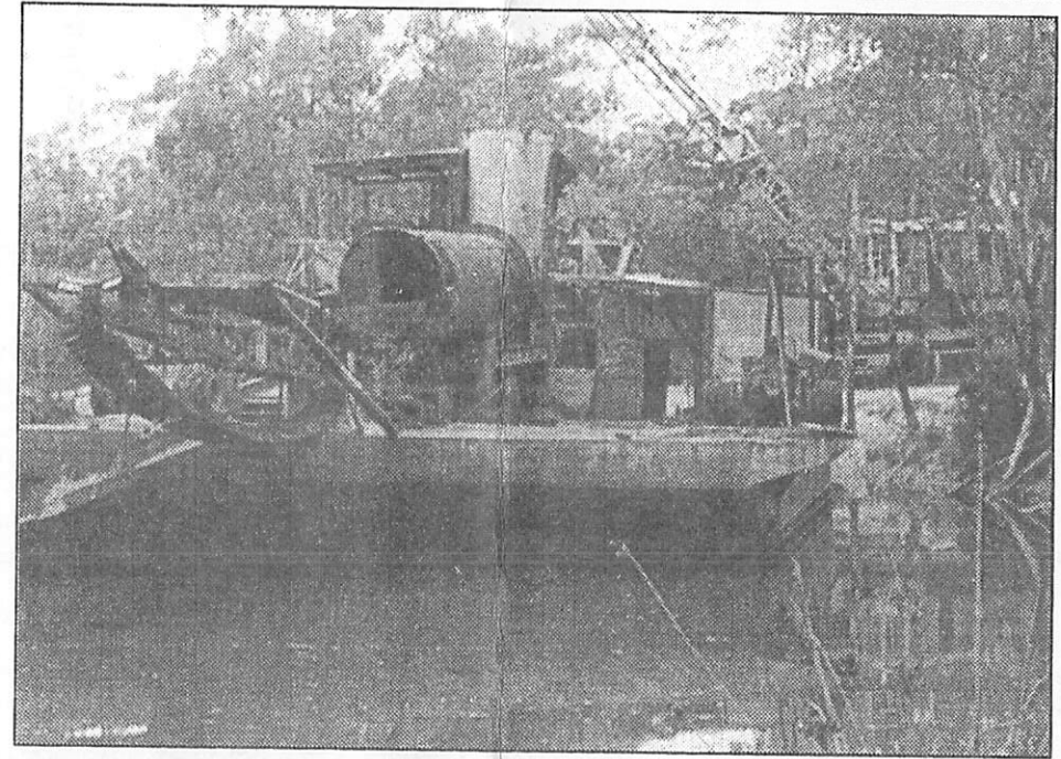
The dredge at Porcupine Flat was made there on site from parts cannibalised from throughout Victoria; the pontoons it floats on from the Strangways dredge, the buckets and other essentials from Bright and Harrierville in the north east.
