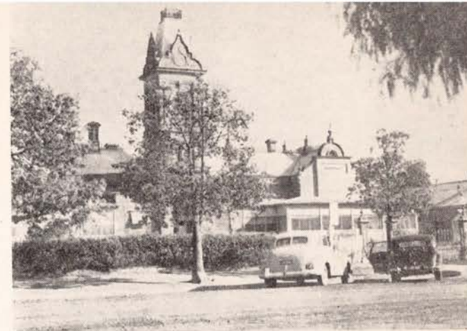
THE SWAN HILL DISTRICT HOSPITAL
