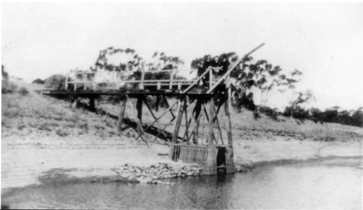
Old Jetty showing drawing arm for water supply for Tarnagulla
