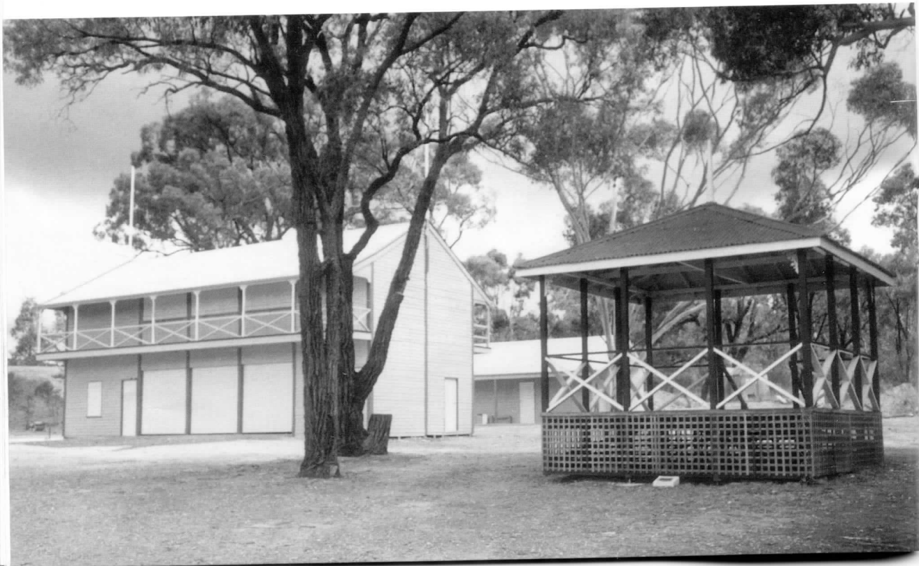
Band Rotunda and Pavilion showing new toilet ammenity in background
