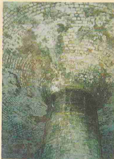
Vaulted roof in Tower 64
