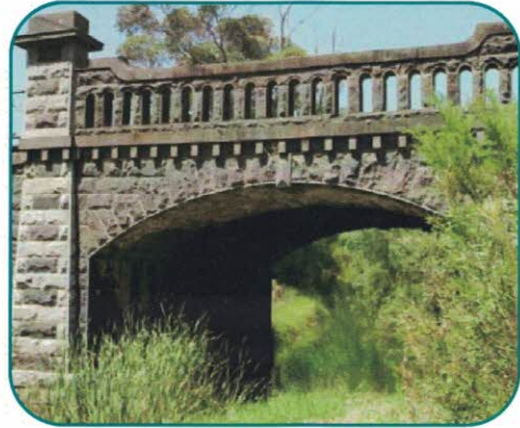
Bluestone and granite bridge Westmeadows
