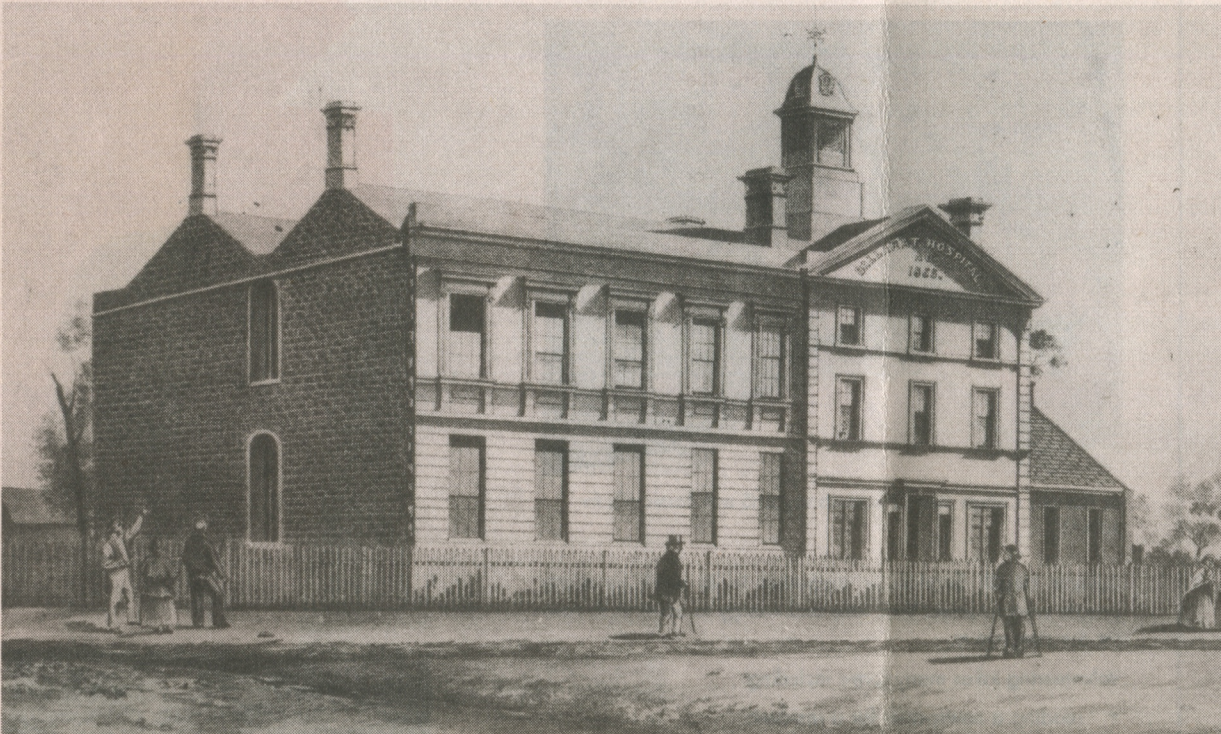
A sketch of the Ladies Wing built in 1858. It was named the Ladies Wing in tribute to fair fundraisers, however female patients were still housed in the tiny north wing.
