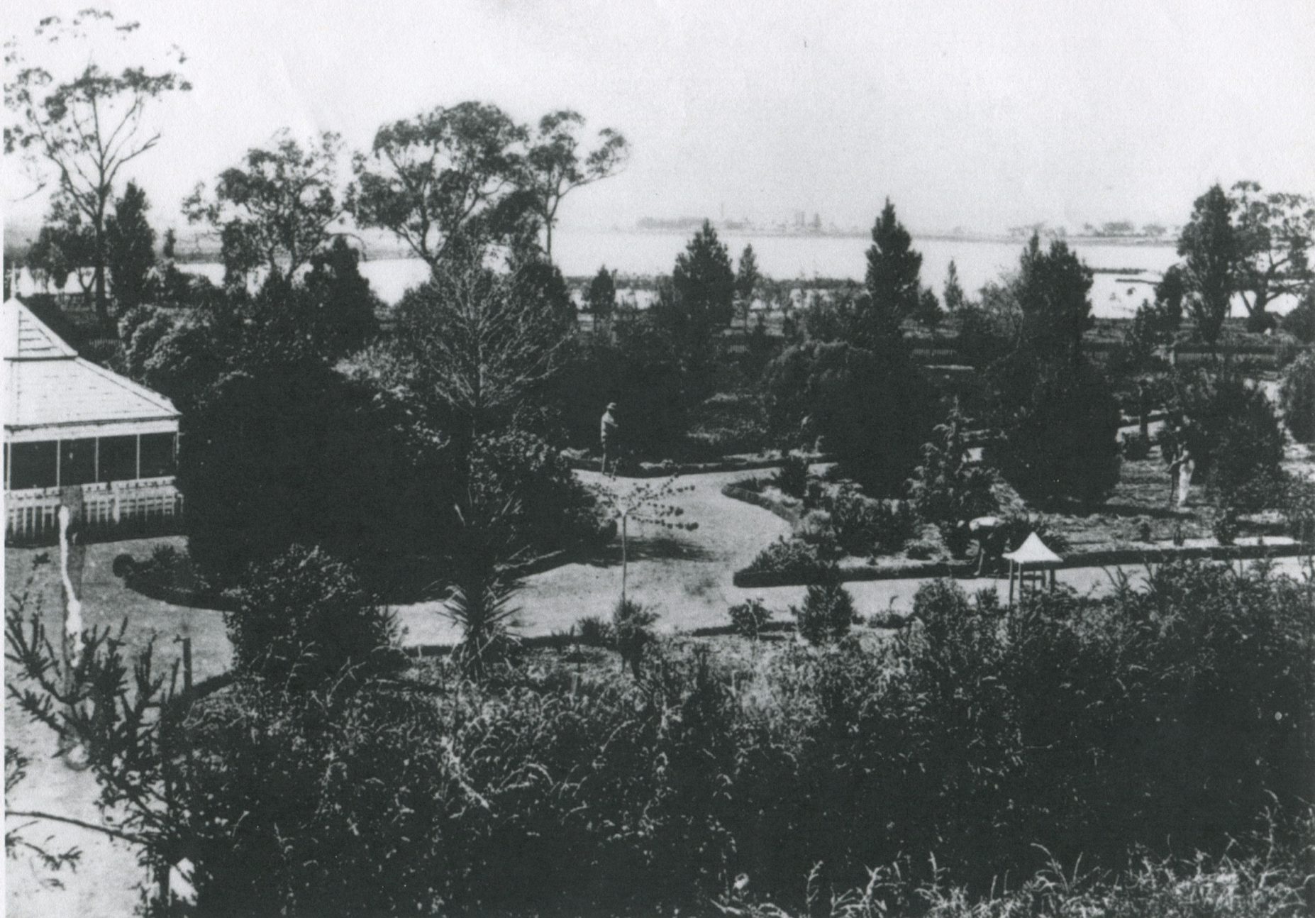
301 BALLARAT GARDENS TAKEN FROM ABOUT WHERE THE STATUARY PAVILION IS NOW SITUATED.
