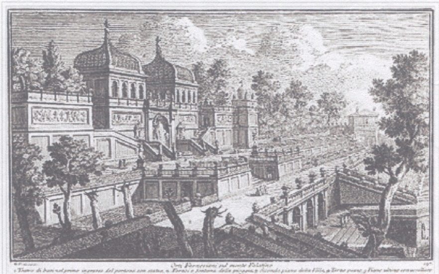
1761 engraving by architect Giuseppe Vasi from book 10 of his series of vedute (views) of Rome, showing the Farnese Gardens on Palatine Hill in Rome at that time. The ground floor entrance is at right, and the twin domes are above the aviaries on the third floor of the structure.
