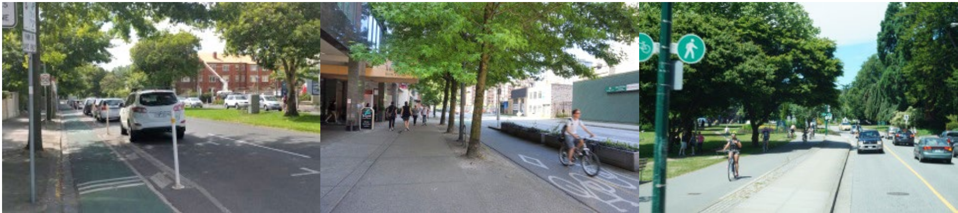
Images: Protected cycleways physically separate people cycling from vehicle traffic. Protected cycleways can be developed using incremental approaches that allow for rapid roll out of low cost networks followed by improvement over time to all ages, all abilities standards.
