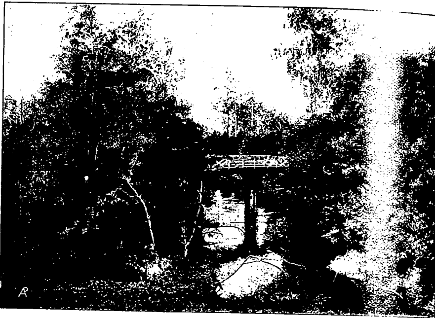
ROOKE'S BRIDGE, NEAR HEALESVILLE.
