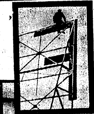
JUST A "SIGN OF THE TIMES" was the removal of the name from the top of the Ford plant in Windsor, Canada, which was dismantled so that the steel framework might be broken up into scrap iron. Some idea of the size of the sign and amount of steel salvaged is gained from the fact that the letters were 10 feet high, making up the name of the Company, stretching 400 feet along the Detroit River. The steel has now been melted down to make vehicles of war, and possibly may be in some of the engines reaching the Ford Co., Australia, where war vehicles of all kinds are being built.
