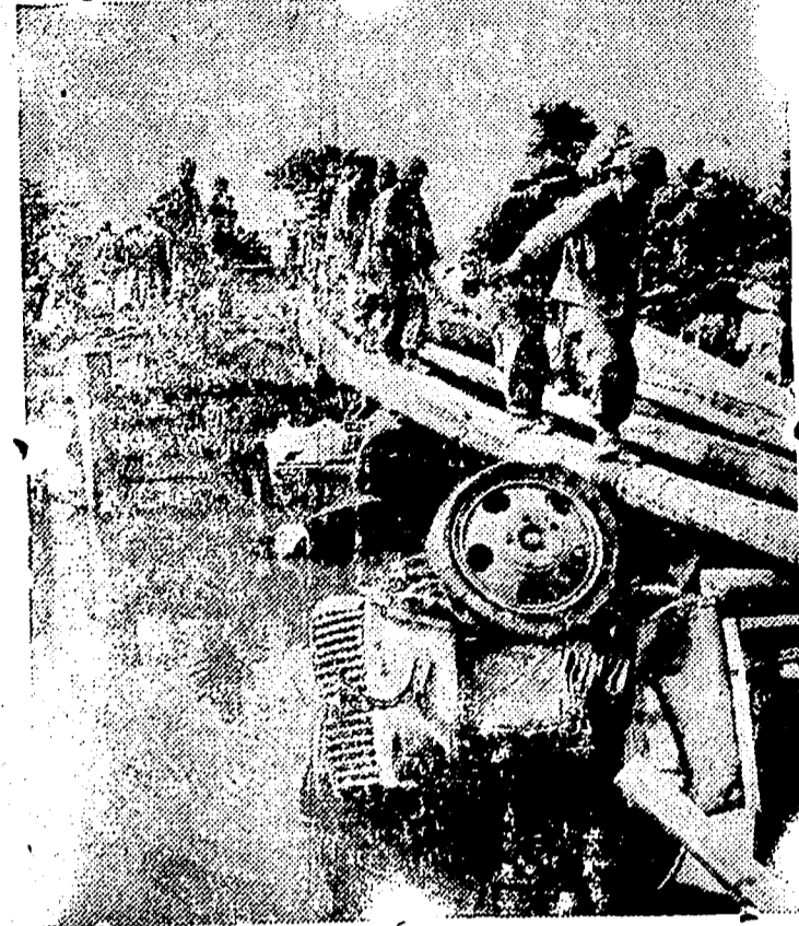
U.S. INFANTRY UNIT BUILDS LUZON BRIDGE. —U.S. Office of War Information Picture.
