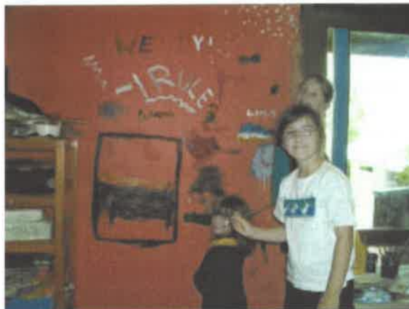
Annie, Bridget and Wendy prepare the back wall for demolition
