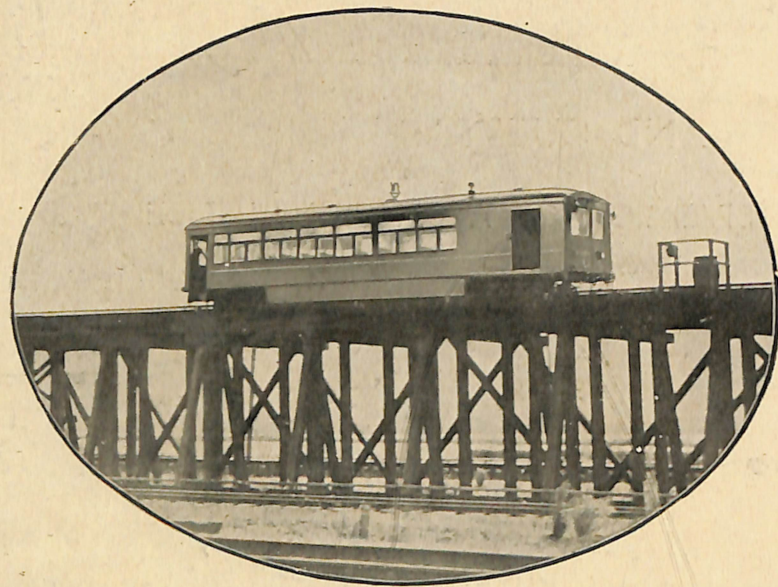
Showing Car on Grade on Trestle. Grade South, 1100', 2.27 percent. Grade North, 815', 2.34 percent.
