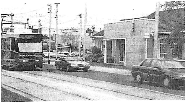
EAST PRESTON TRAM DEPOT
