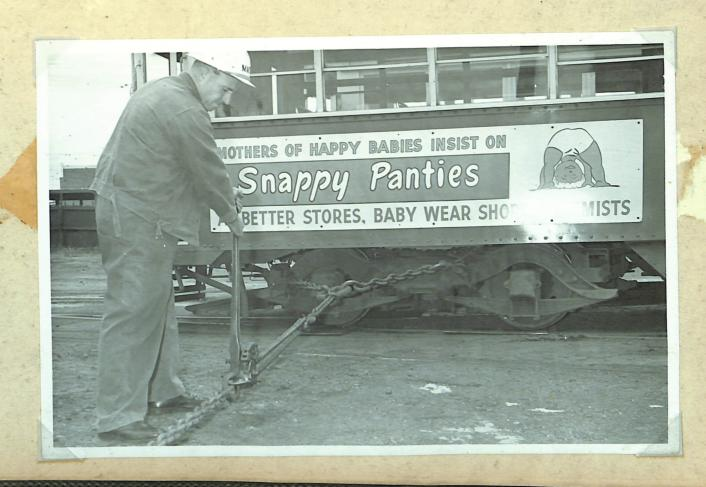
Two traction type hoists are used for emergency work, the Tractel hoist, shown in figure 2 and the Reco hoist shown in figure 3.
