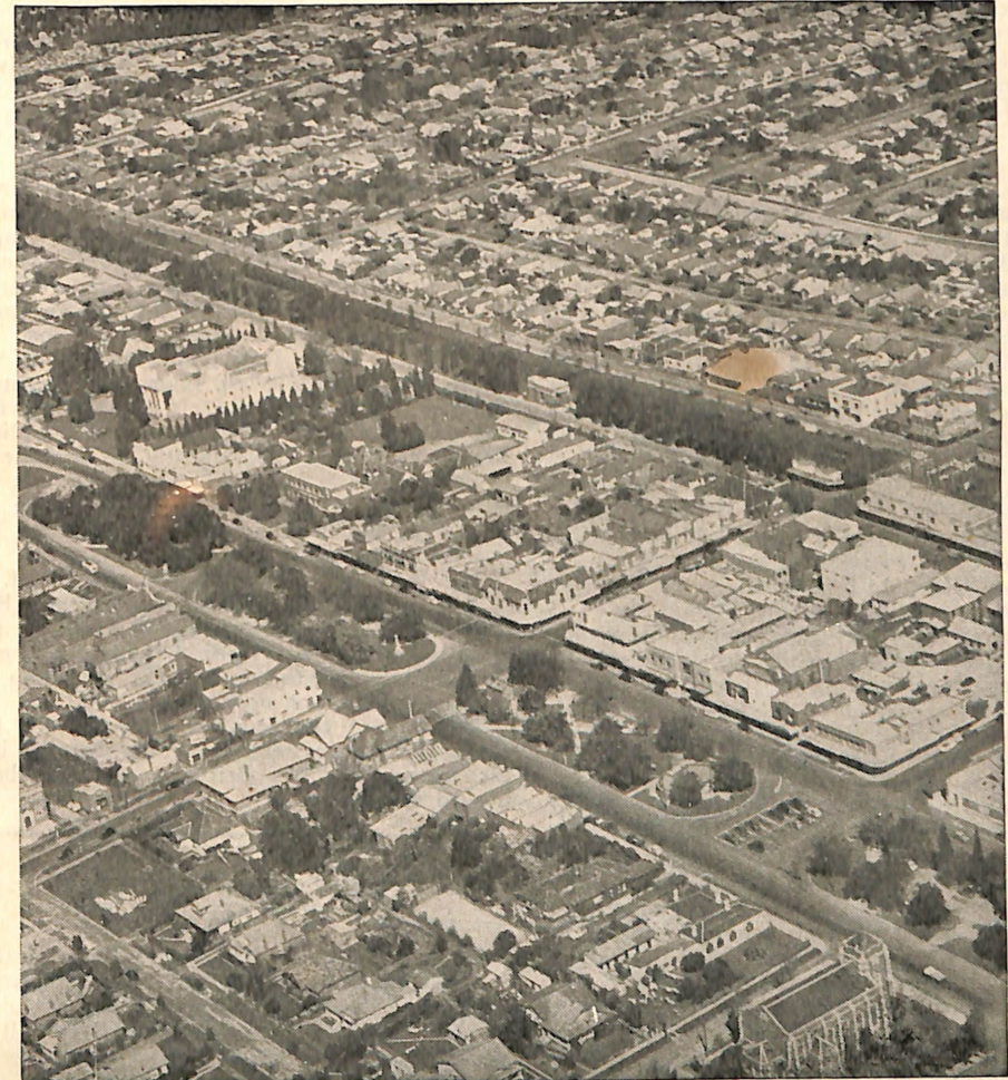
Box Hill shopping centre today. The terminus was near the lower left of the picture, where Station Street enters Whitehorse Road, the latter being the wide, divided highway.
