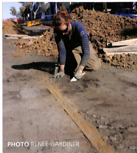
Above: A section of Melbourne's original cable tramway was exposed during roadworks in North Melbourne in May 2007.
