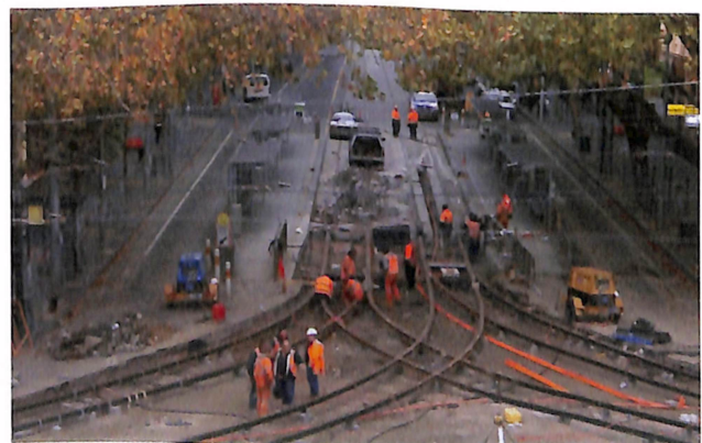
New tracks allow Route 48 trams to turn from Spring Street into Collins Street.
