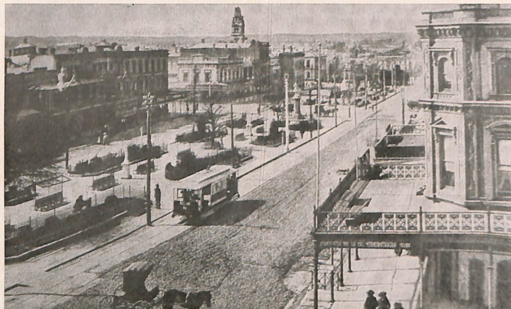
An early electric tram grinds along an unusually deserted Sturt Street.
