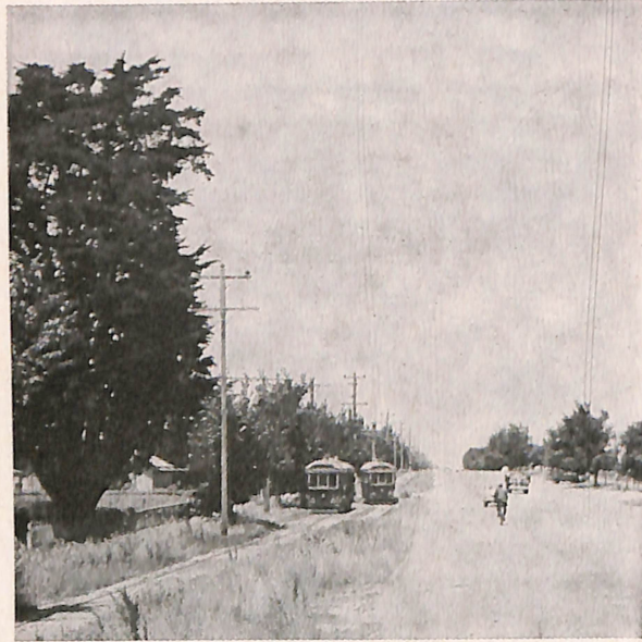
The side-of-road rural atmosphere of the Sebastopol route is shown as two cars pass on the crossing loop.
