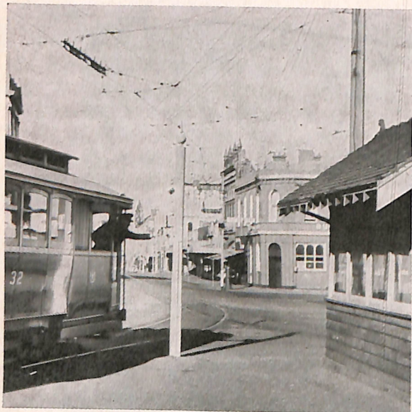
The small pole-mounted box allows the motorman to select the correct signal light setting for his passage into Bridge Street to the Victoria Street or Mount Pleasant routes, or to shunt and return along Sturt Street.
