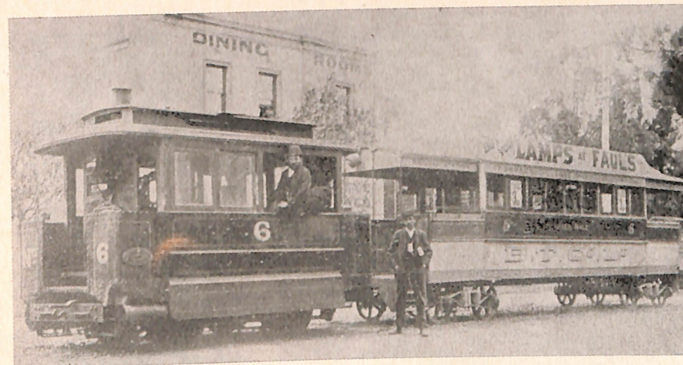
Phoenix-built motor No. 6 and trailer No. 5. The 3d. fare advertised on car windows was pre-payable by ticket printed green on white paper.
