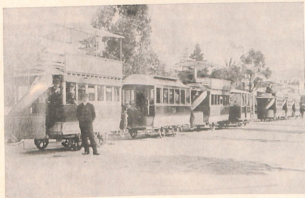
Trailers provide additional accommodation for crowds from the station. Single deck cars are former steam trailers, the smaller being an "umbrella" car.
