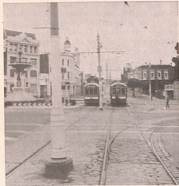
Nos. 2 and 25 pause before rumbling over the 1903 concrete-based cobble stoned track of the central city area.
