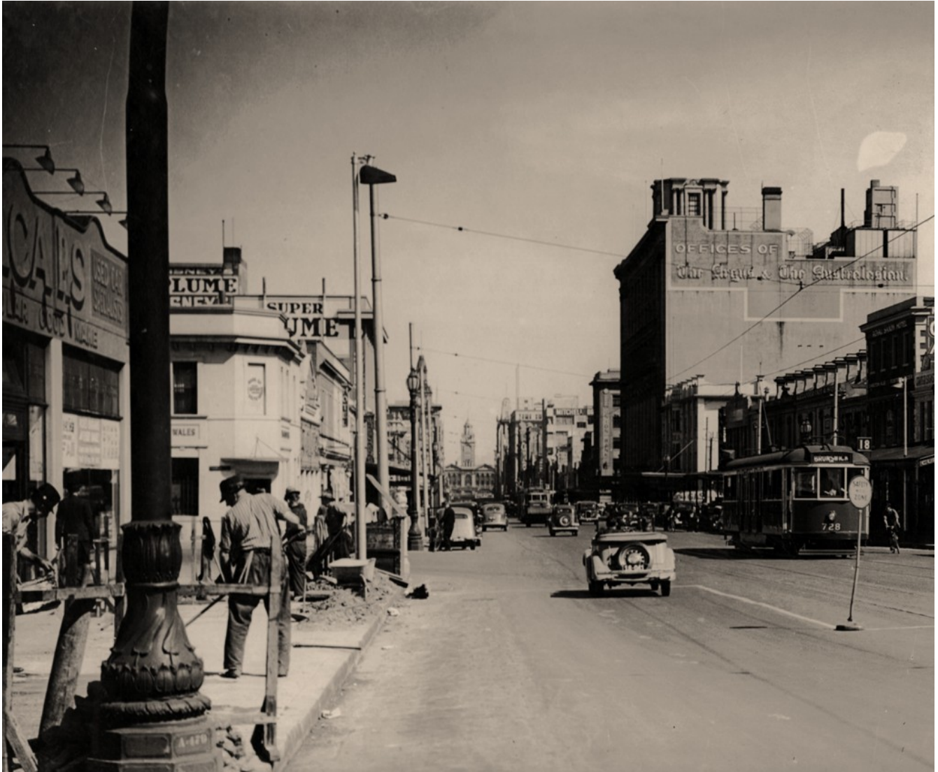
Looking south along Elizabeth St from north of the Franklin St intersection, circa 1950. W5 728 is on a route 18 short working to Brunswick. The office of 'The Argus' is the tallest building in view. Photo donated to FOHTD Collection by Ron Scholten.
