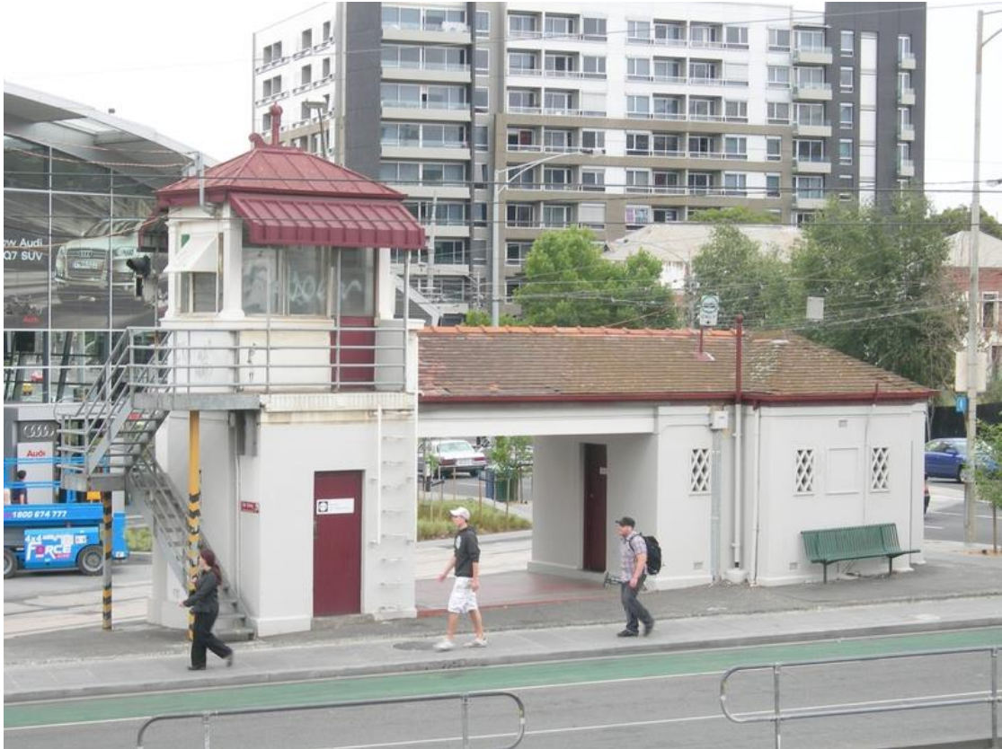
Figure 4: The Tramway Shelter pictured in 2008 showing the added steel staircase.
