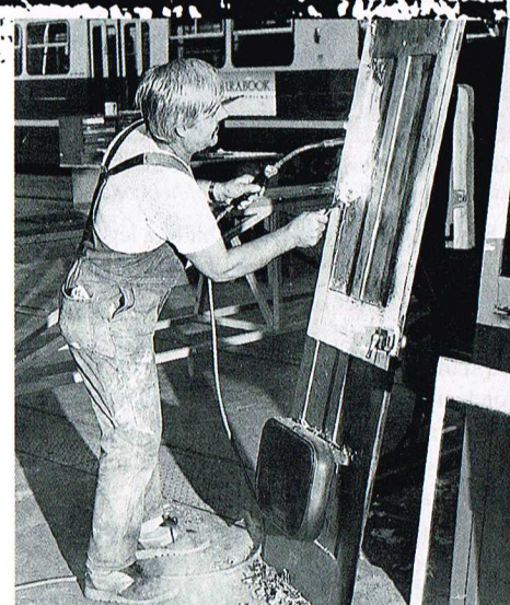
The driver's door is removed from the vintage tram to enable Vehicle Painter, Con Vlahakis to strip the paint
