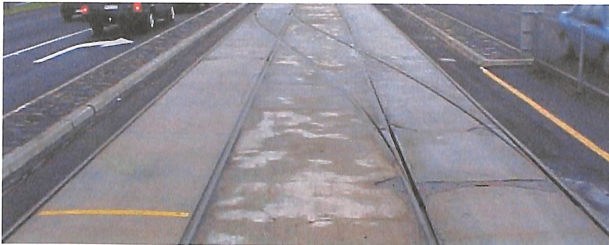
Fouling mark on left track for crossover
