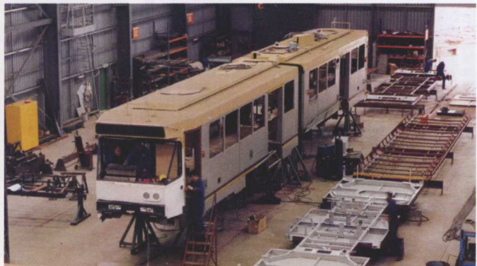
One of the prototype articulated B-class trams under construction at Comeng Dandenong.
