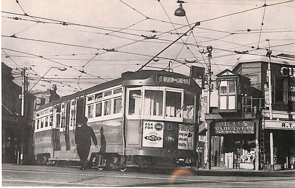
L class No. 104, designed for the Prahran and Malvern Tramways Trust and completed for the M&MTB in 1921, displays its Brill 79E trucks and extra width to good advantage as it short turns at St. Kilda Junction in November 1967 under the watchful eye of the point controller's box on the right, before reconstruction of this important intersection had begun. Ward Collection
