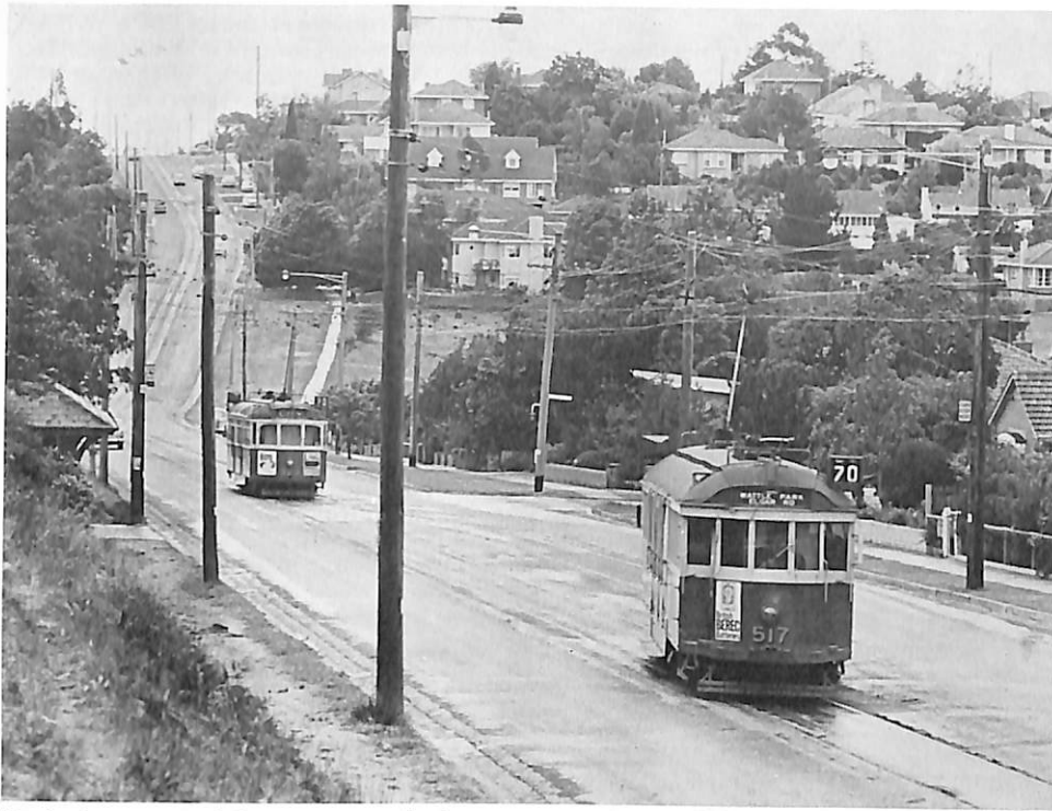
The furthest extent of the tram system is the outer, eastern end of Route 70 Wattle Park, some 8 miles from the City, seen here prior to its recent double-tracking. The vehicles which have just looped (passed) include No. 923 an SW-6 and No. 517 a venerable 1928-built W-2. To the left is Wattle Park, owned and operated by the M&MTB in the manner of early American electric trolley amusement parks, with some of 517's stripped brethren being provided there for children to play on.
