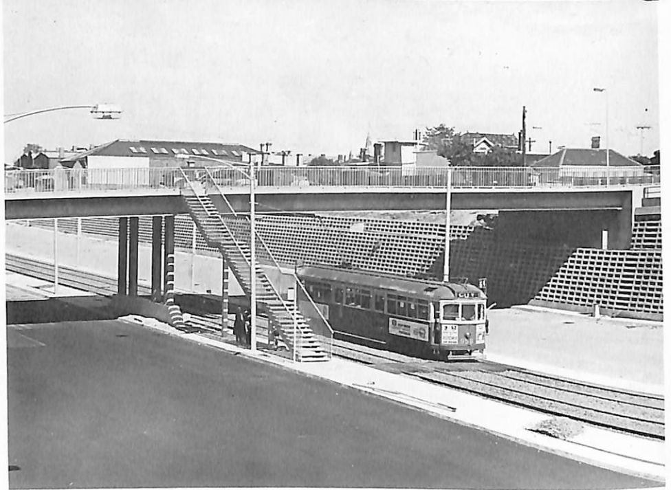
A view of the new median strip operation built as part of the complex split-level tram and road interchange at St. Kilda Junction. Although No. 958 is a post-War enclosed car, 40 to 50 year old W-2 class cars are quite common on this stretch of Routes 5 and 64 providing a quaint contrast between the old and what is hopefully to become the new standard for reserved track tram operation. Ward collection
