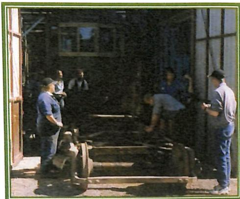
*The Bendigo crew removing the temporary trucks from under L 103 prior to reinstalling the overhauled trucks.*
