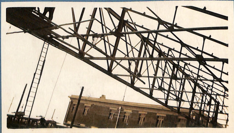
View Showing Trusses at entrance. Traffic offices in background.
