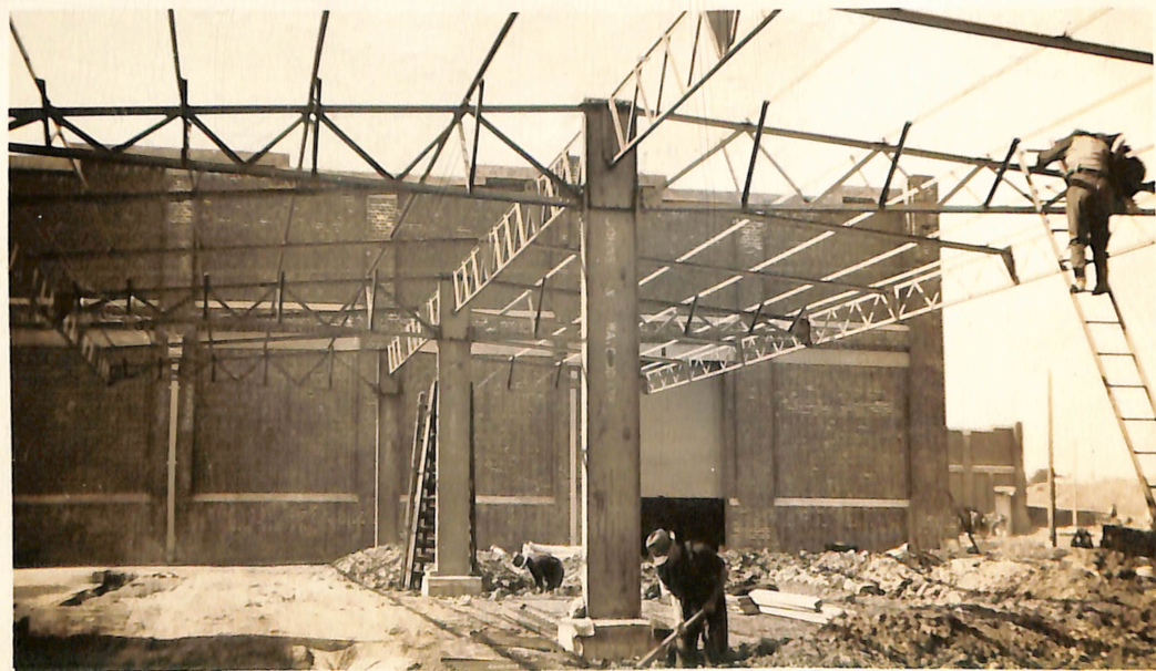
Canilever type sheds for seasoning Timber
