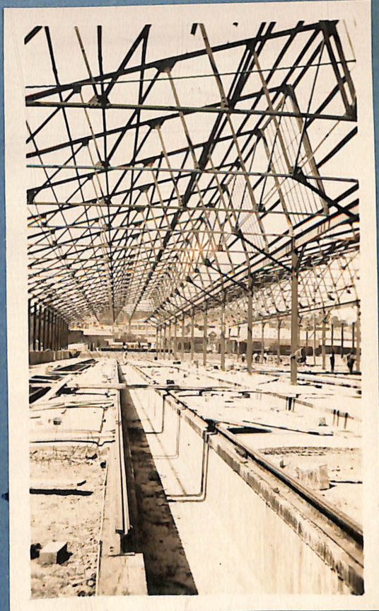
View Showing Roof Construction and track pit.
