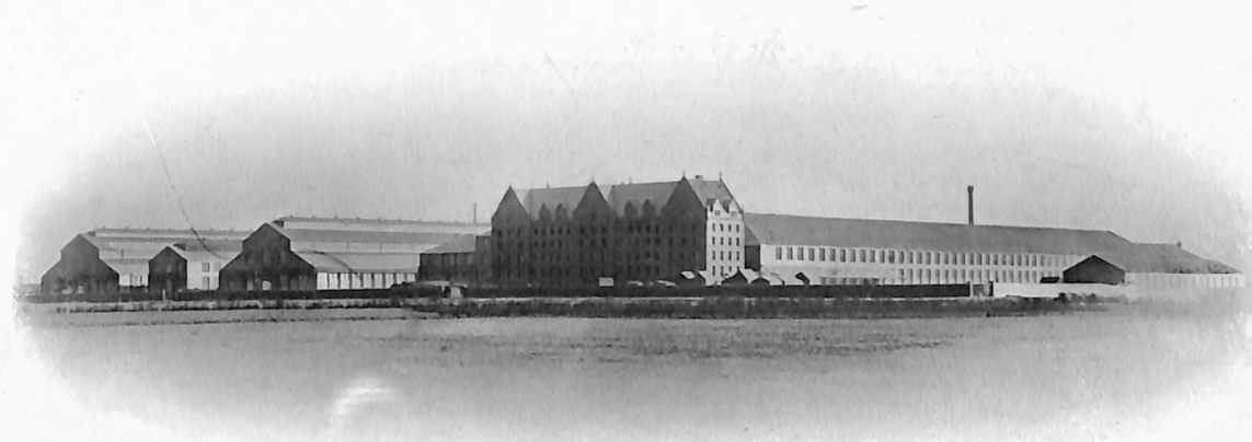
Westinghouse Works, Manchester, England.
