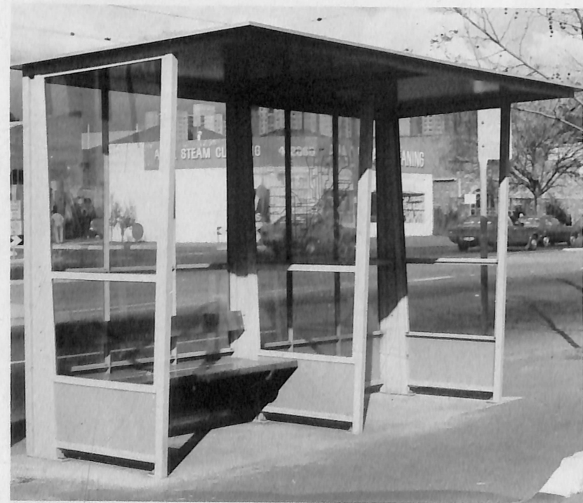
The steel framed 'double' modular shelter which was first developed in the late 1960s.
