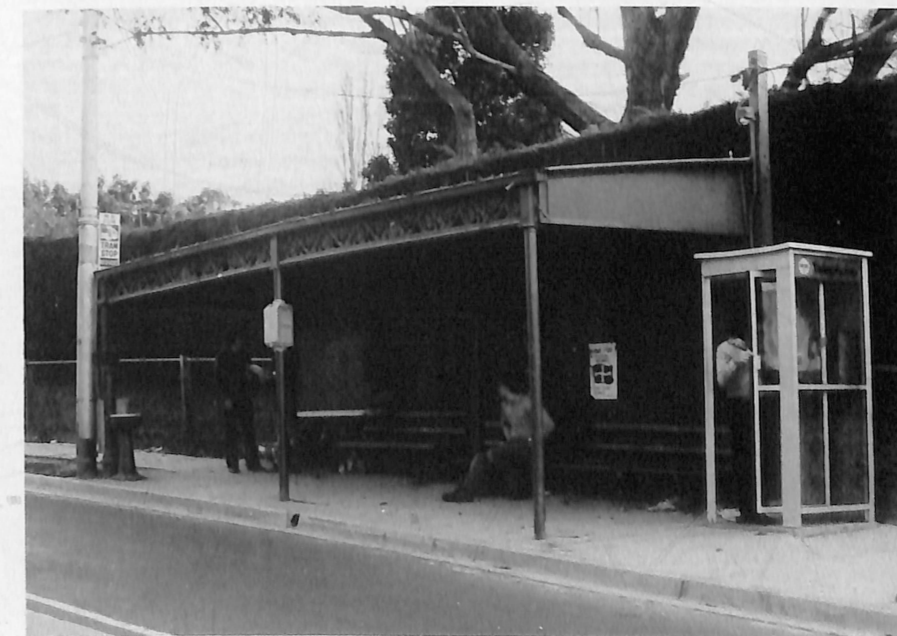
One of the first tram shelters erected by local authorities. These are maintained by the MTA's Civil Engineering Branch.
