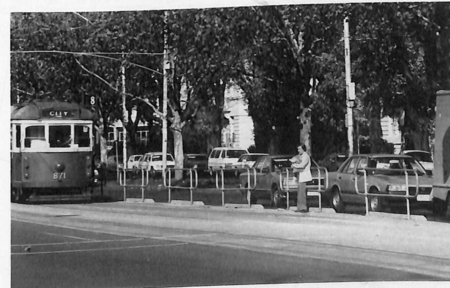
A view of the older style of safety zones which features the distinctive tubular steel railing.
