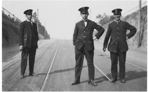
Trammies in Barkers Road Cutting in 1922. Photo: William Simpson
