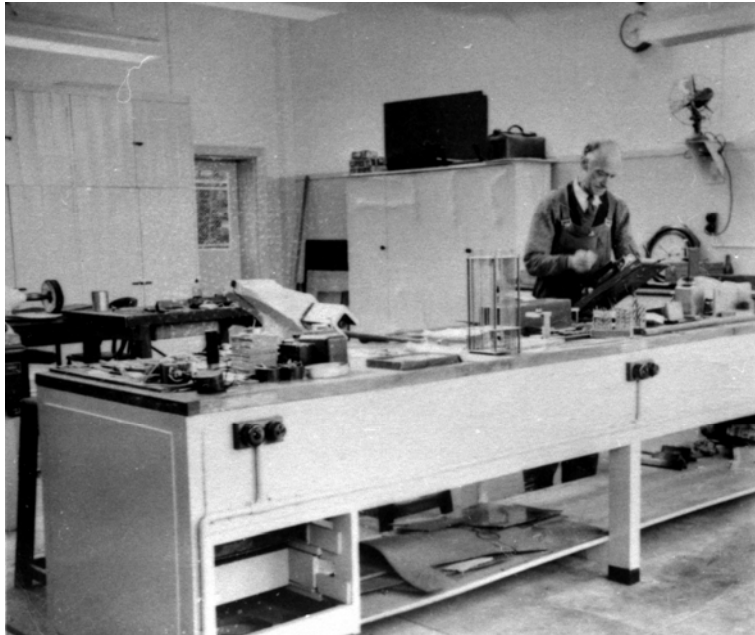
William Simpson at work in the Electrical Shop at Preston Workshops.
