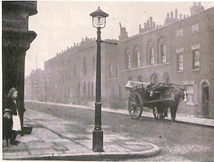
"G.E.C. Patent Lantern, Switch and Fuse with Robertson Carbon Filament Lamps" in one of the streets of Poplar, London, 1900.
