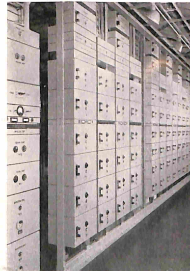
Electronic equipment on national trunk telephone circuits, enabling twelve conversations to take place simultaneously over one pair of wires.
