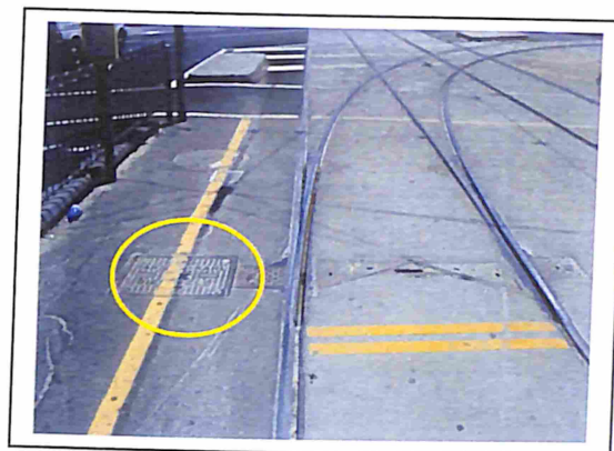
Turnout with Automatic Points
