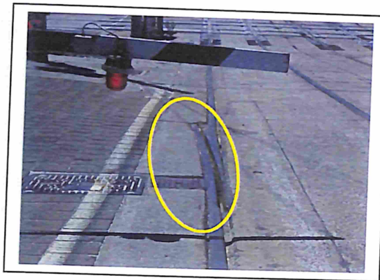
Tram Catch Points at Level Crossing
