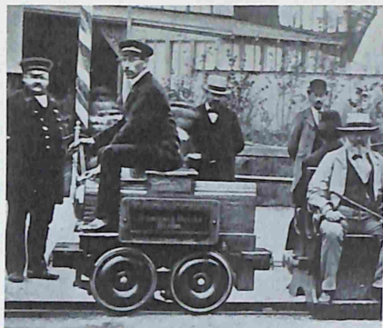
The first electric locomotive, constructed by Werner von Siemens 1879
