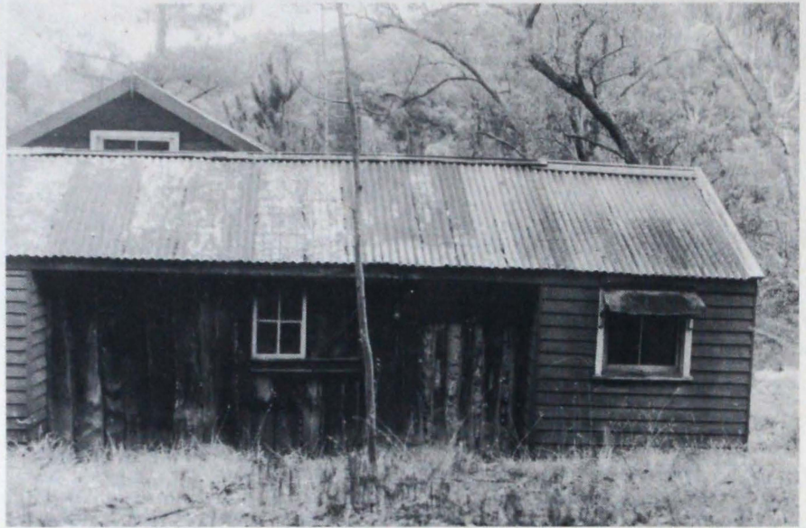
The wall that provided the clue to the discovery: the only external sign of anything unusual.
