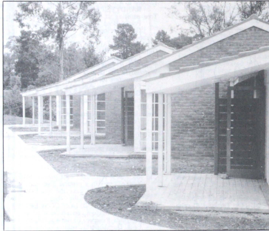
These flats for the elderly are almost finished down opposite Stiggants Reserve.
